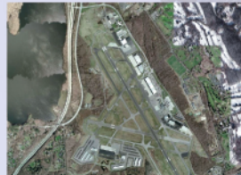
HPN - Westchester County Airport
